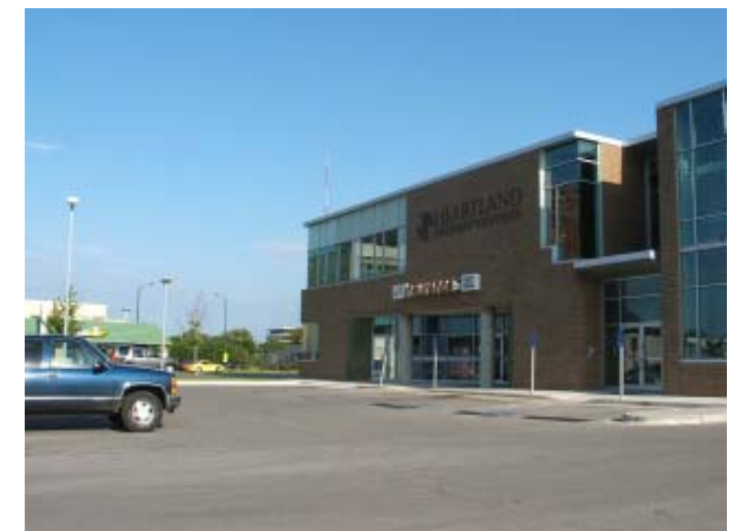
Bad: Door opens to parking lot at Linwood & Main
