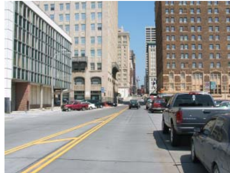
Good: Re-done Baltimore Ave.
