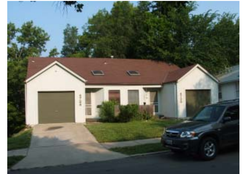
Bad: West Plaza neighborhood duplex
