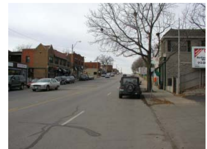
Bad: Westport Road @ Wyoming
