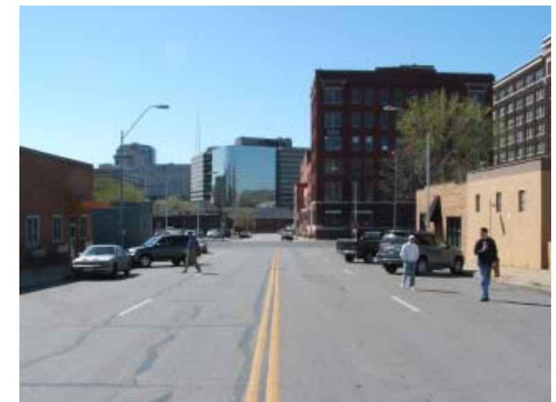
Bad: Baltimore Ave before the makeover
