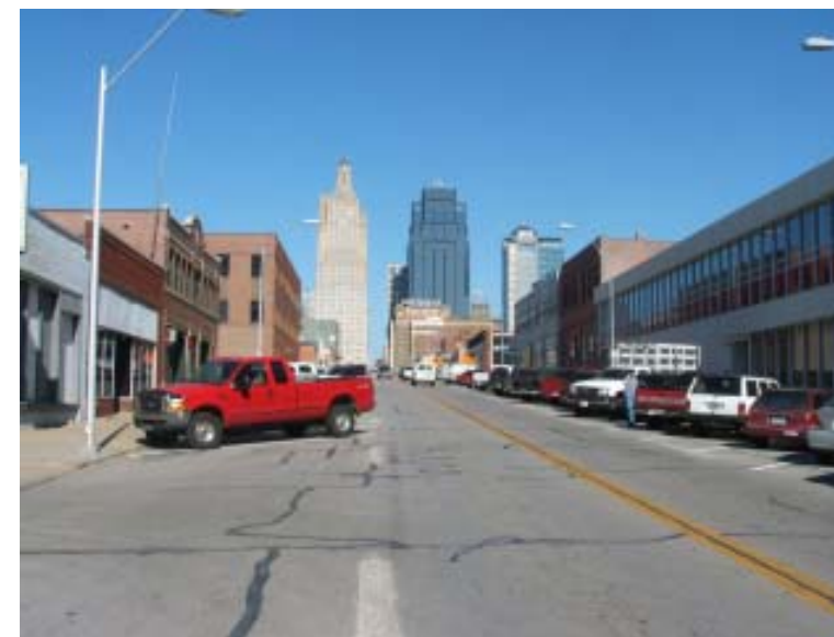
Good: Baltimore Ave with angled parking
