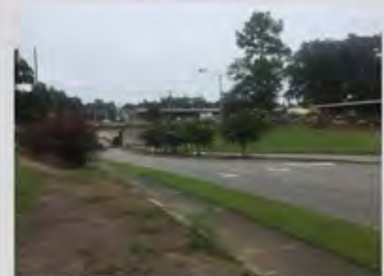
Hansell Street appears to have a great deal of excess lanes and paved area, and could be improved quite easily with some simple landscaping and design techniques.
