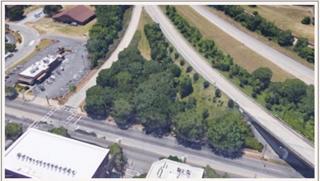
Aerial of MLK, Jr. Blvd. at the Flyover
