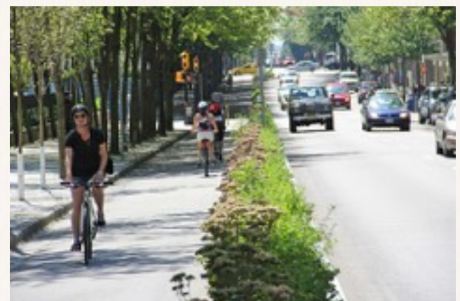
A 2-way protected bike lane
